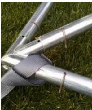
8' long loop strap is "noose" wrapped around the frame at corners and tees
